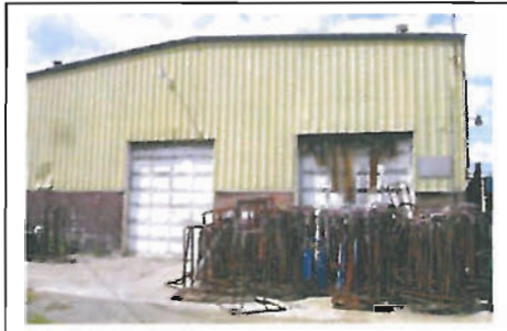
Drive-In Doors East Side
