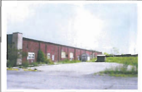
Southern Elevation Along Rail Line
