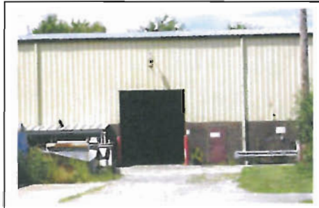
Drive-In Door East Side
